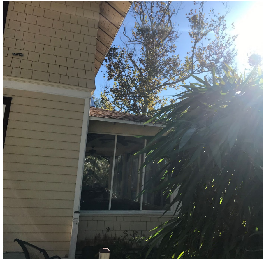
North Elevation: looking south at northwest corner
