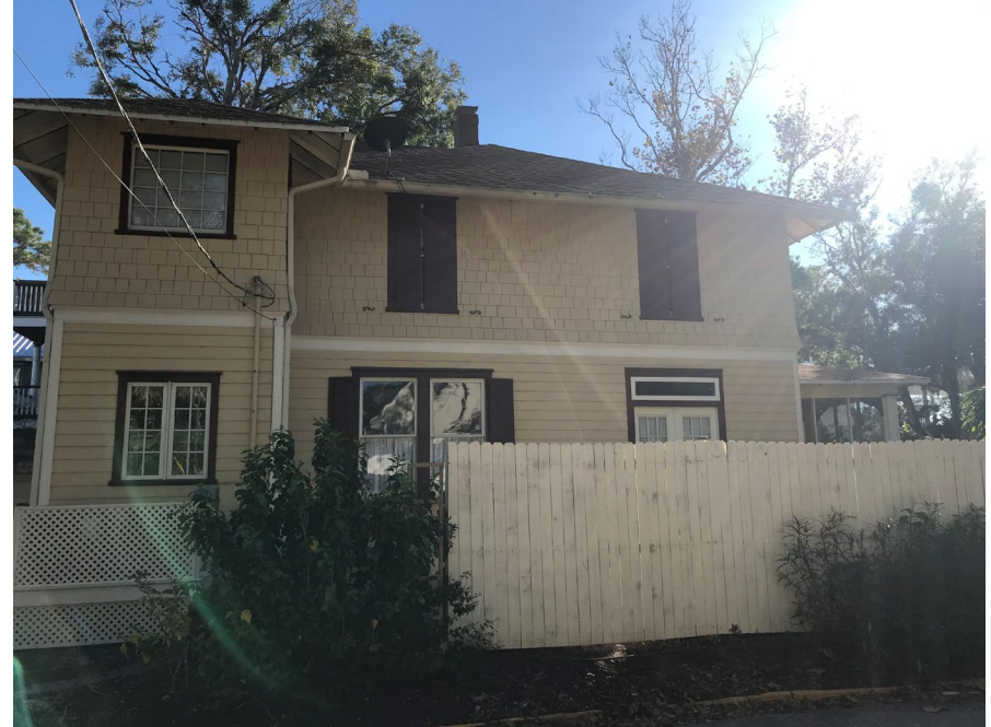
North Elevation: looking south
