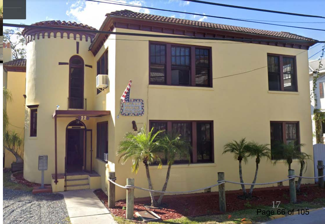
Example of replacement windows:
