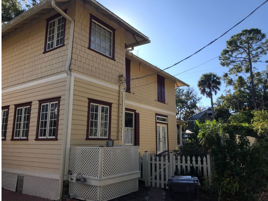
North Elevation and corner of East elevation: looking southwest
