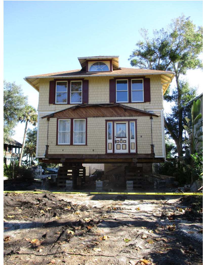
Front Façade / West Elevation: looking east After porch was removed
