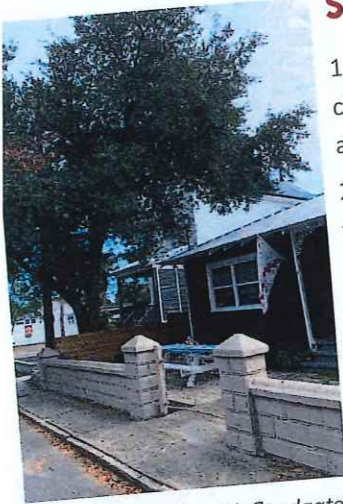
Masonry site walls with floodgates can provide flood protection. Image from ML+H.
