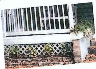
Example of Raised Pier construction with porous skirting (lattice). Image from ML+H.
