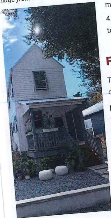
A low site wall can help to provide flood protection. Also shown is an open "pier system" for the front porch. Image from ML+H.
