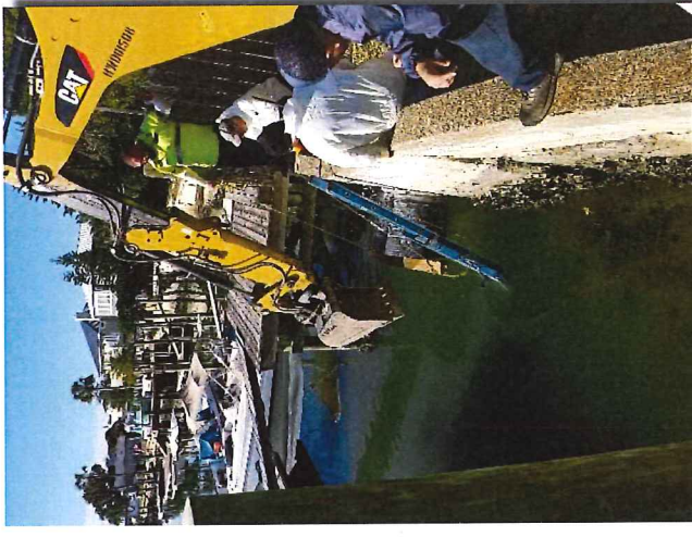
City installation of one-way tidal valve in FDOT outfall
