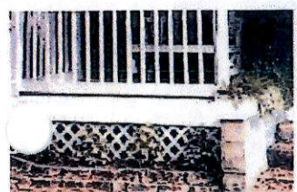
Example of Raised Pier construction with porous skirting (lattice). Image from ML+H.
