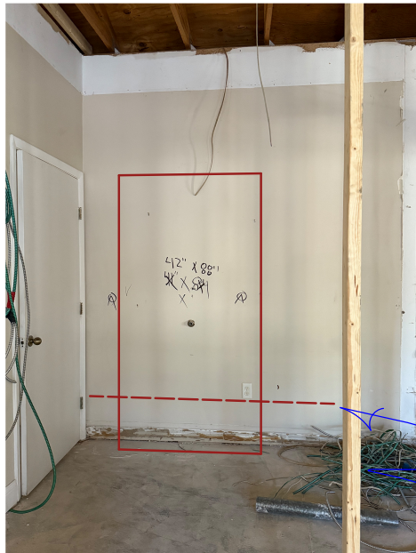
INTERIOR ARCH CUT TO PROPOSED DOORWAY
