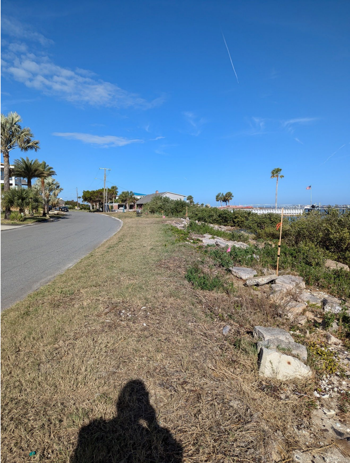
Proposed wall alignment staked by surveyor. Orange flag represents the top of the proposed wall.
