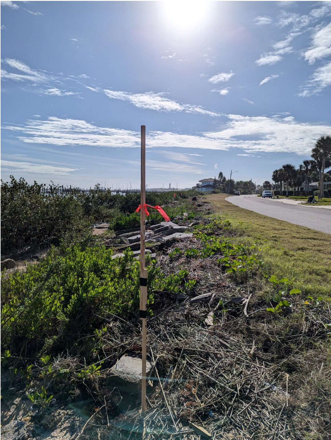
Proposed wall alignment staked by surveyor. Orange flag represents the top of the proposed wall.
