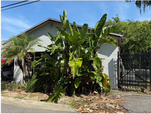
SOUTH WALL AND EAST CORNER
