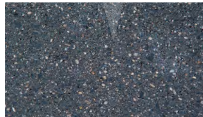
TARMAC CHECK HERE
