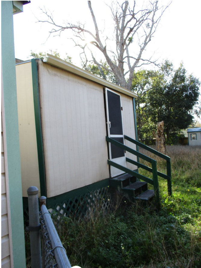
North elevation of rear addition: facing southwest
