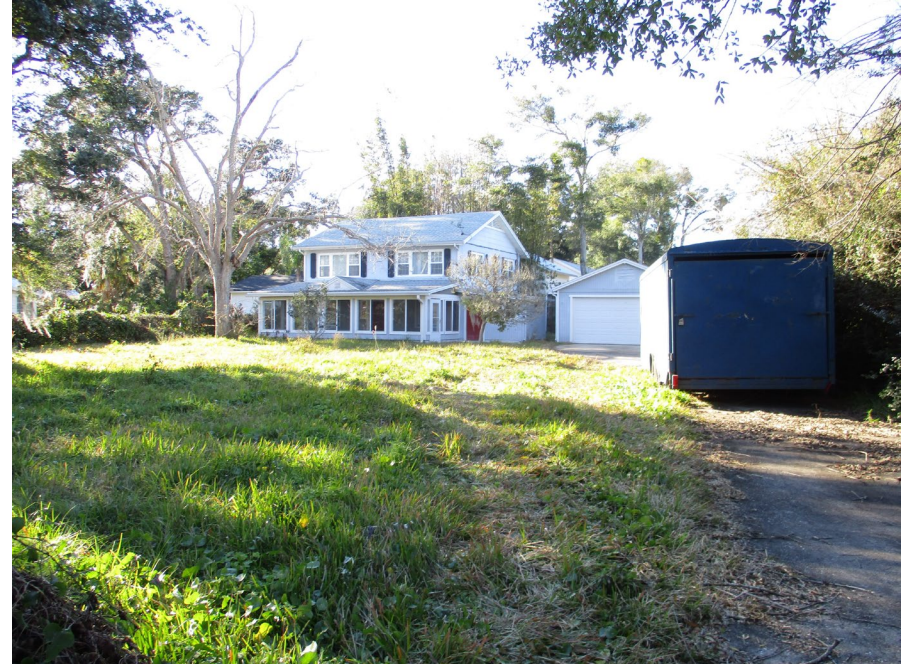
Front Façade (Facing Northwest)
