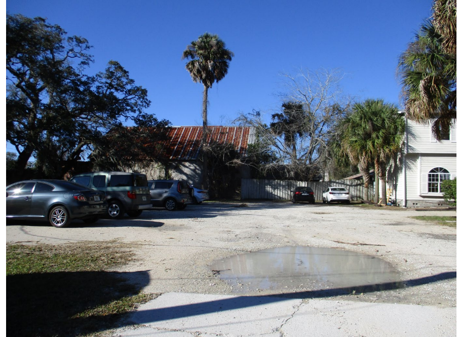
Behind the building, looking North
