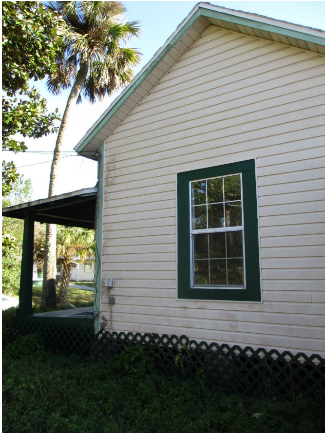
North Elevation of main block
