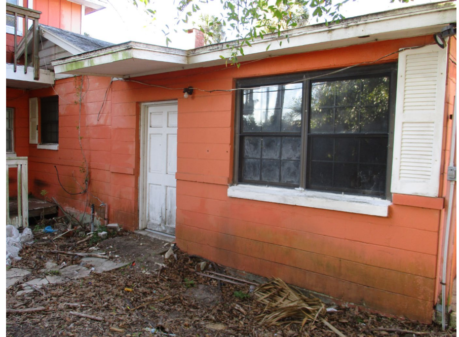
South Elevation / rear of house
