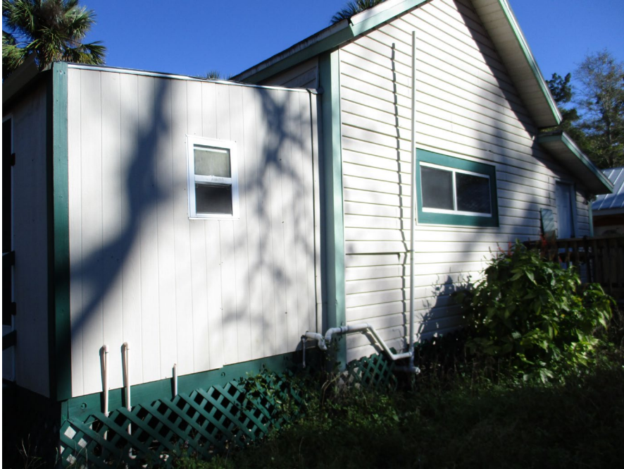
Rear of house: West Elevation
