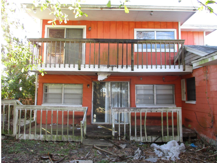
Rear addition: looking West
