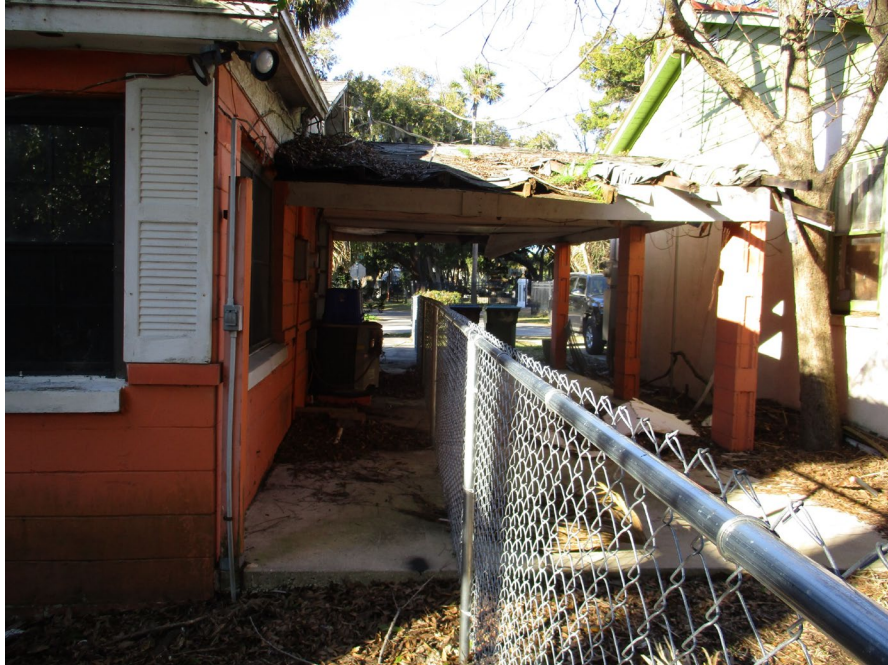
Carport on east end of house and South Elevations
