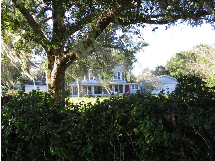
Front Façade / South Elevation (Facing Northeast)
