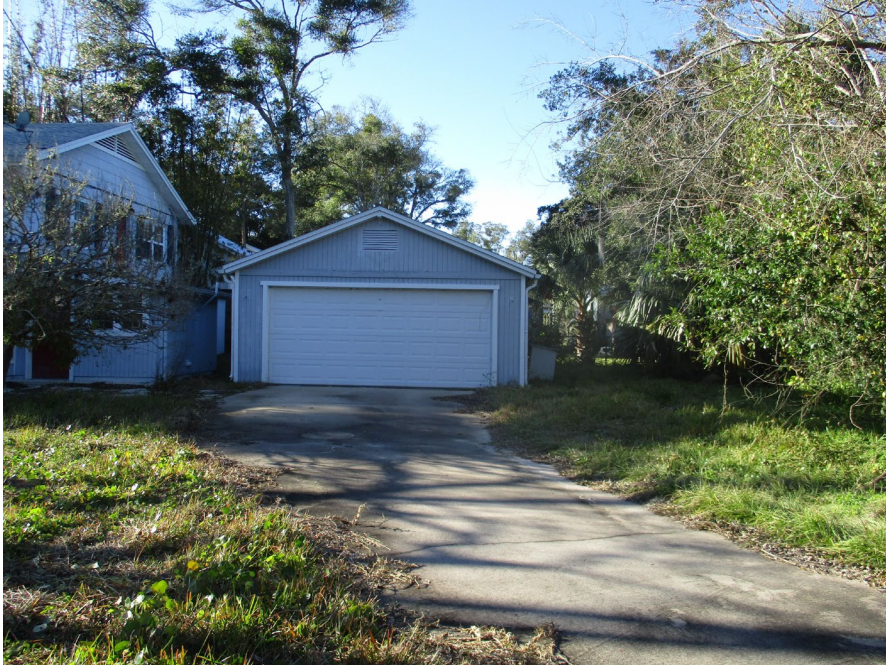
Garage: South Façade
