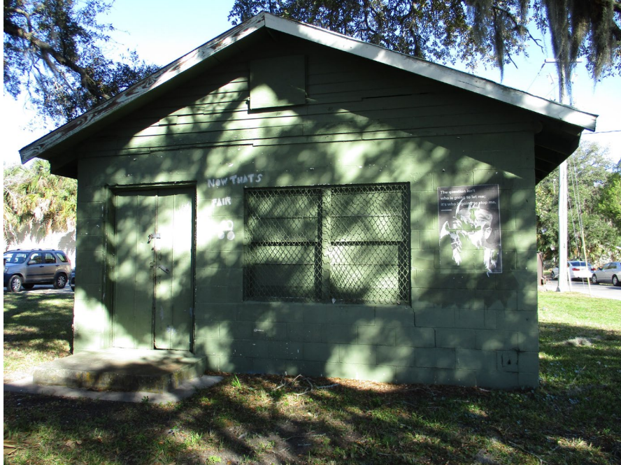
Front Façade / West Elevation
