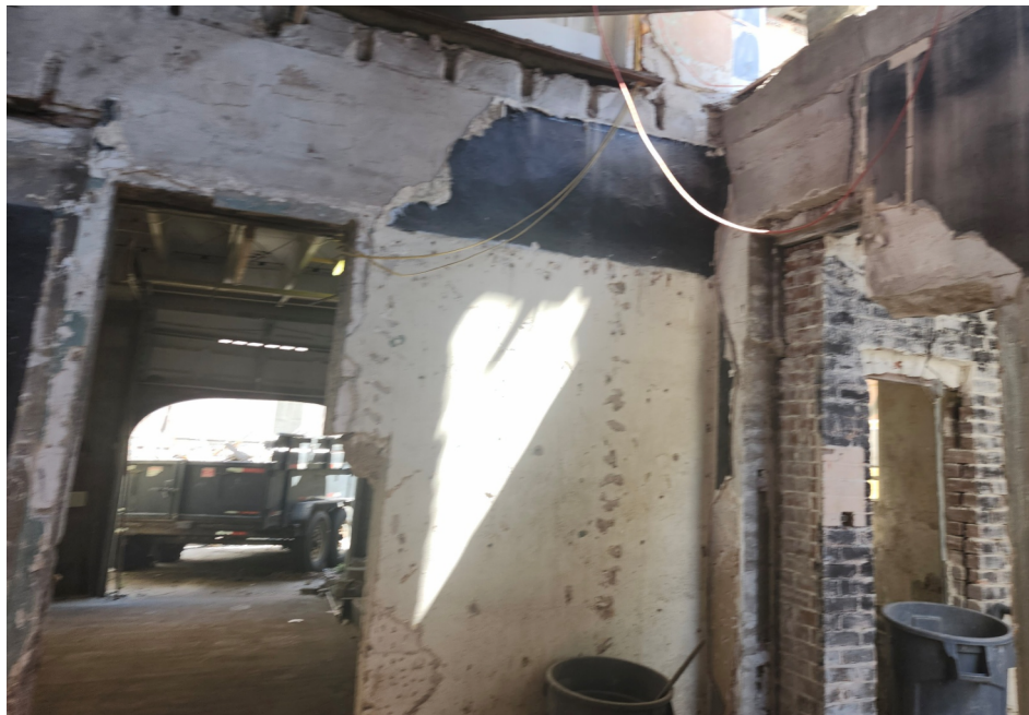
Photograph 2 - Modified Coquina Walls
