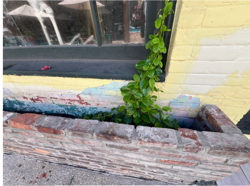
Brick planters to be removed
