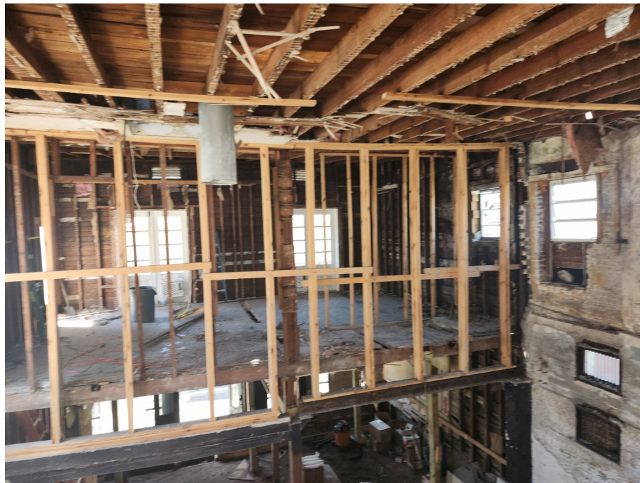
Photograph 4 - Temporary Shoring Supporting Roof Framing
