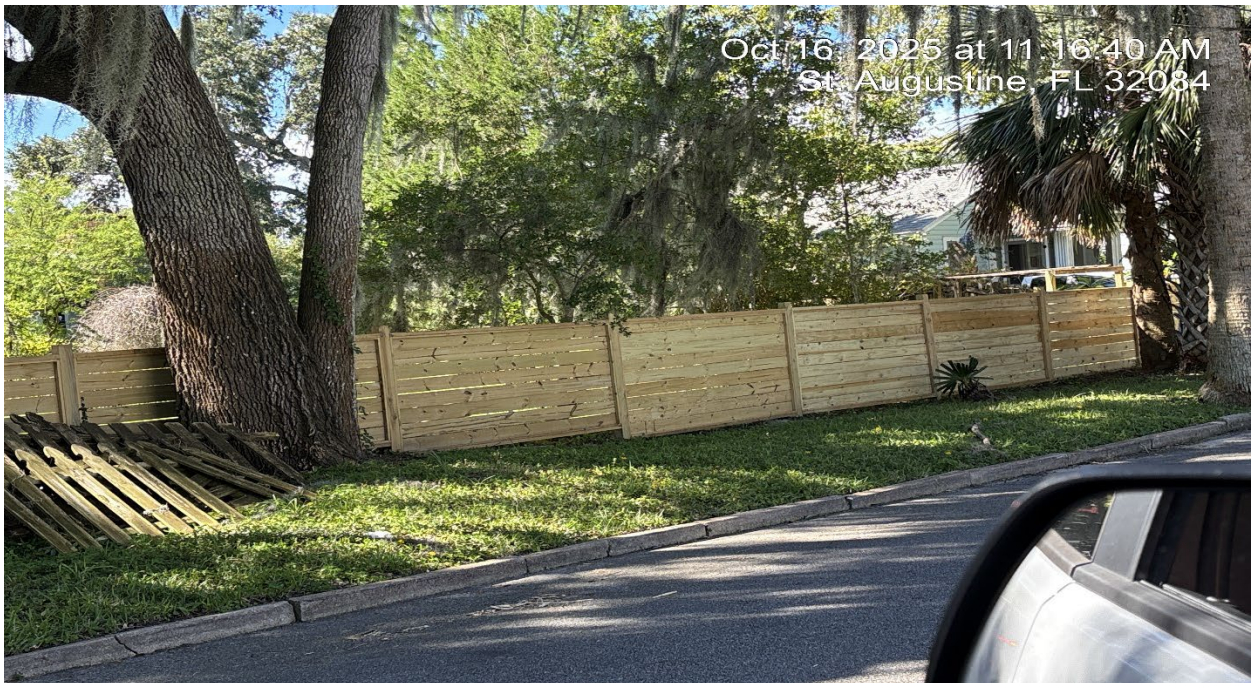
NEWLY INSTALLED FENCE ALONG NORTH PROPERTY LINE
