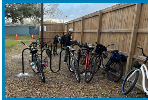
Bike Rack Install
