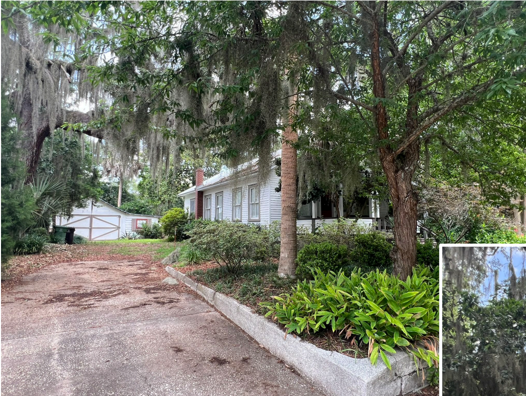
Views of Garage from Sidewalk and Driveway
