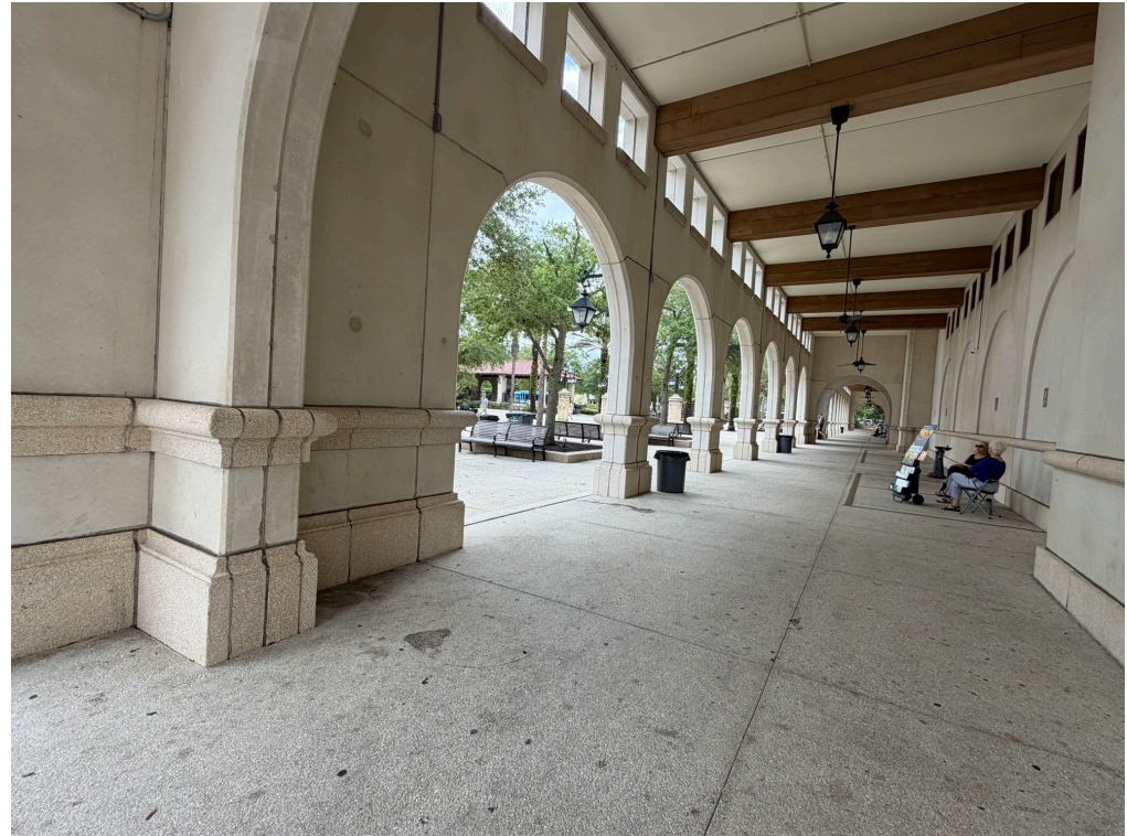
Under loggia of North and East Elevations: facing West Castillo Drive and Visitor Information Center (VIC)
