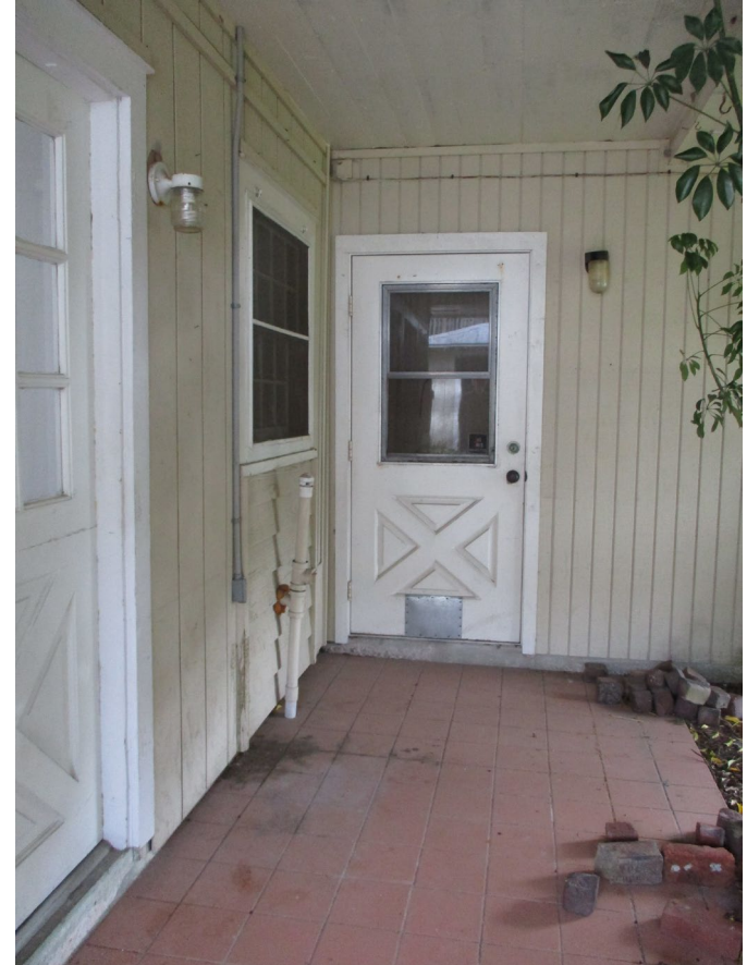
West Elevation and back door to first unit and entrance to second unit on southwest corner
