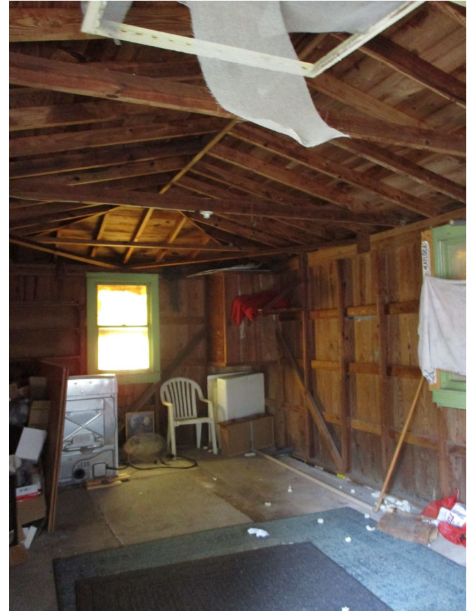
Detached garage to the west side of property
