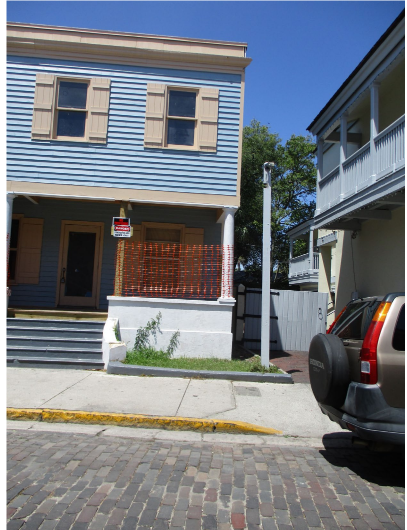
Front Façade / East Elevation and Northeast corner of front porch
