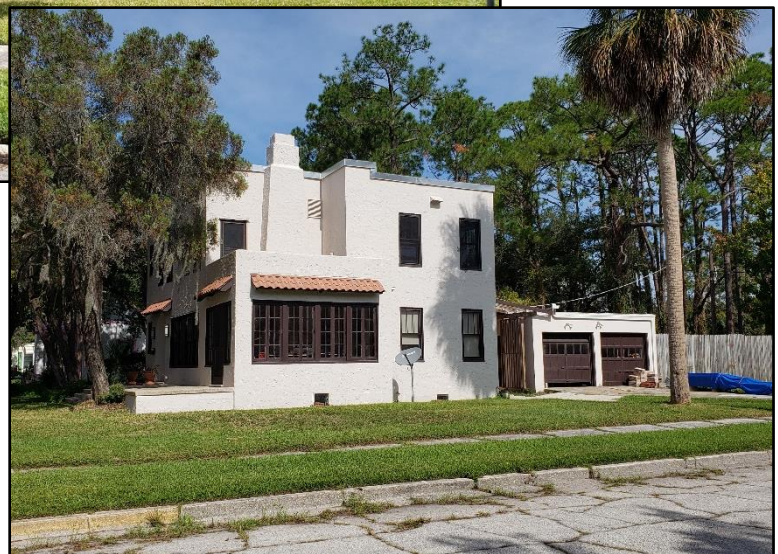
Figure 27. 68 Colon Avenue, side elevation, SJ00642.
