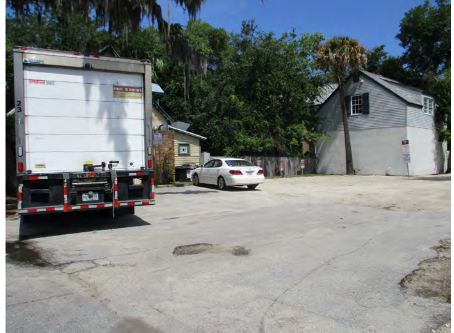
Parking area to be improved with patched paving and ADA striping
