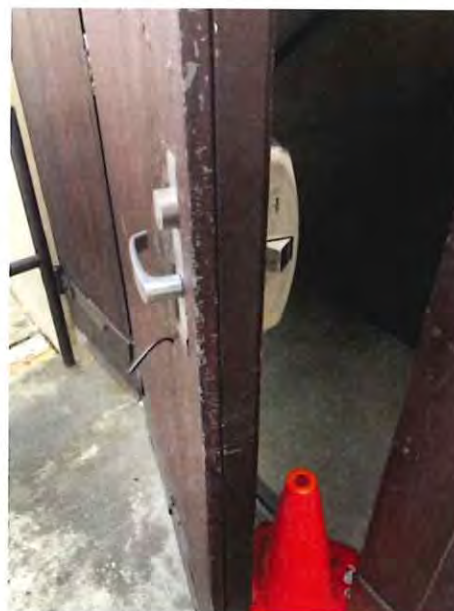
Construction of Exterior Door
