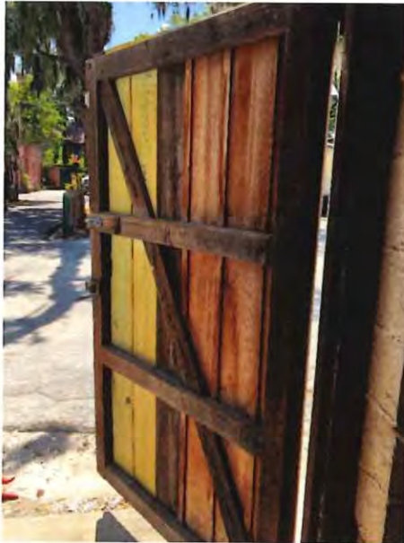
Interior Face of Existing Main Entry Door on West
