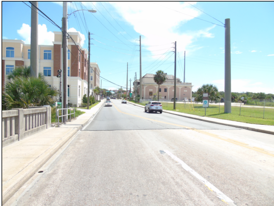
EAST APPROACH TAKEN FROM THE STRUCTURE
