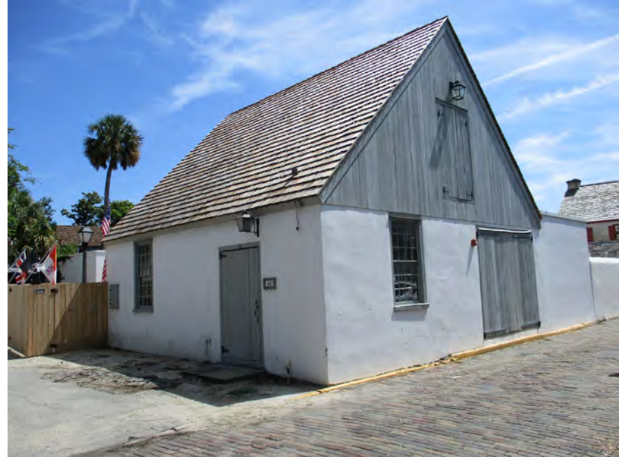
From Cuna Street facing northeast (west and south elevations)
