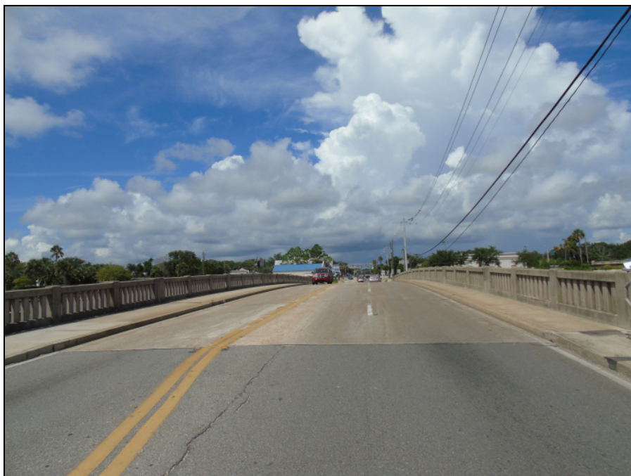
VIEW OF STRUCTURE FROM THE EAST APPROACH
