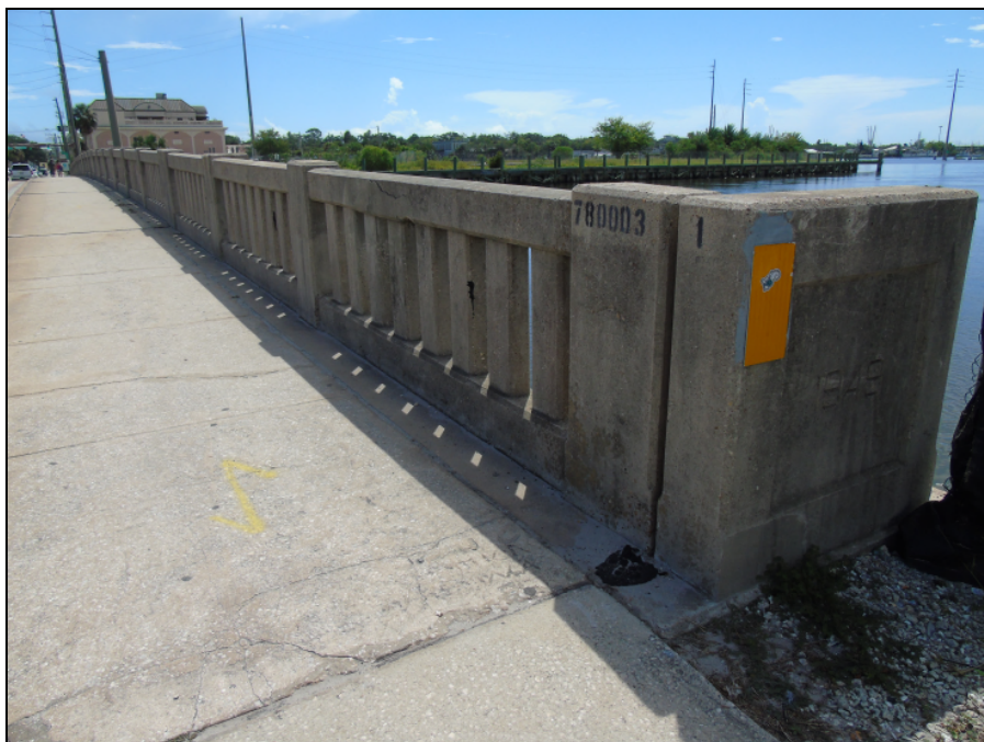
TYPICAL VIEW OF HANDRAIL BARRIERS
