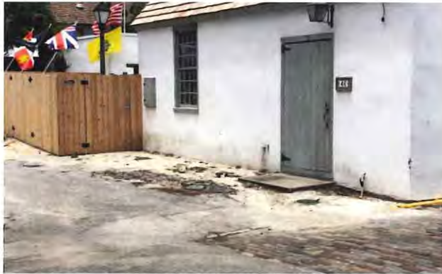
Existing Site Conditions on West Elevation
