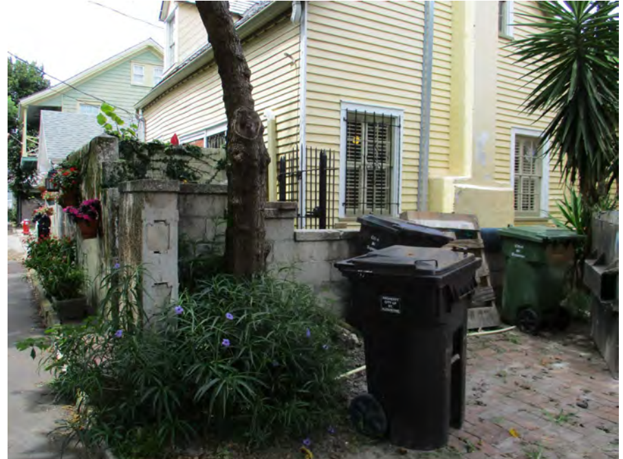
Front Façade / West Elevation and South Elevation with chimney and wall
