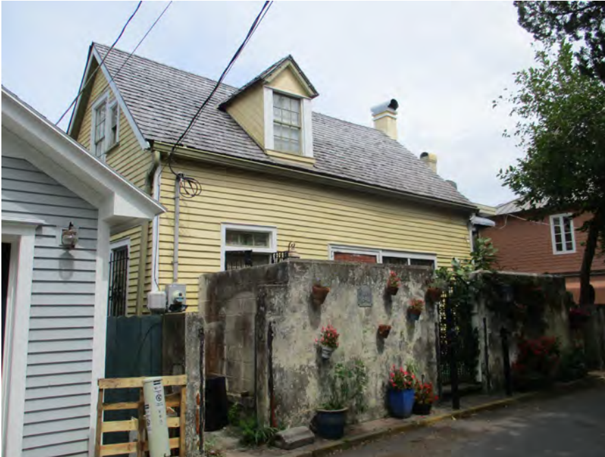
Front Façade / West Elevation with property wall and North Elevation
