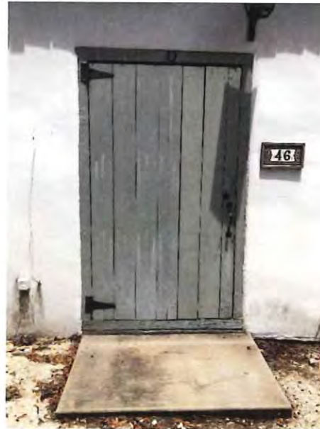
Exterior Face of Existing Main Entry Door on West
