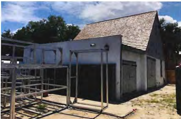
Existing Site Conditions on East Elevation
