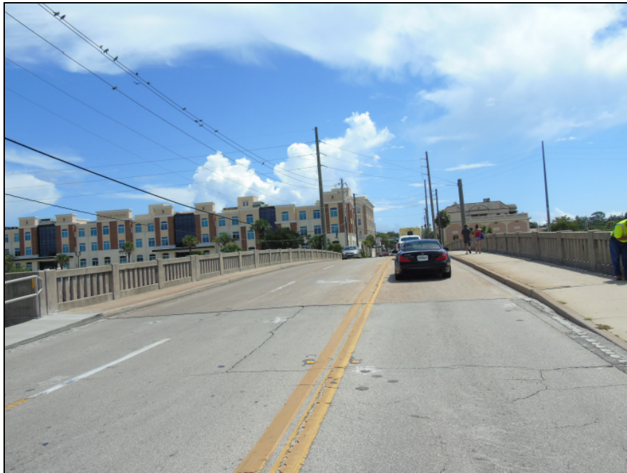
VIEW OF STRUCTURE FROM THE WEST APPROACH
