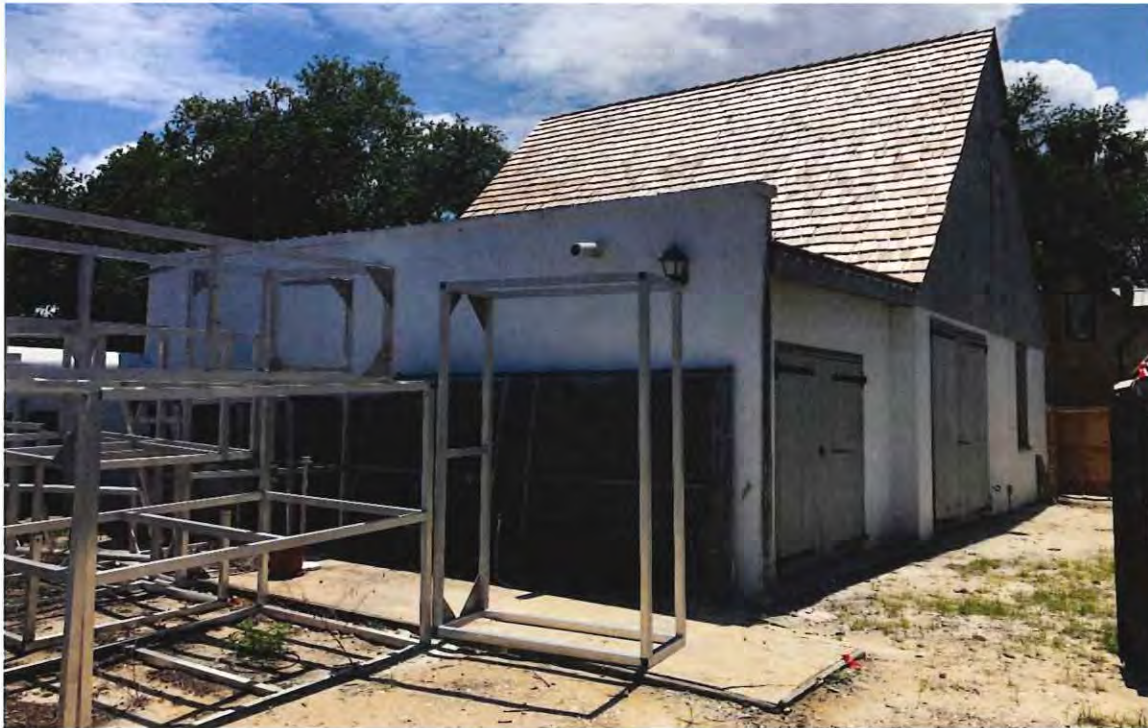
Existing Site Conditions on East Elevation
