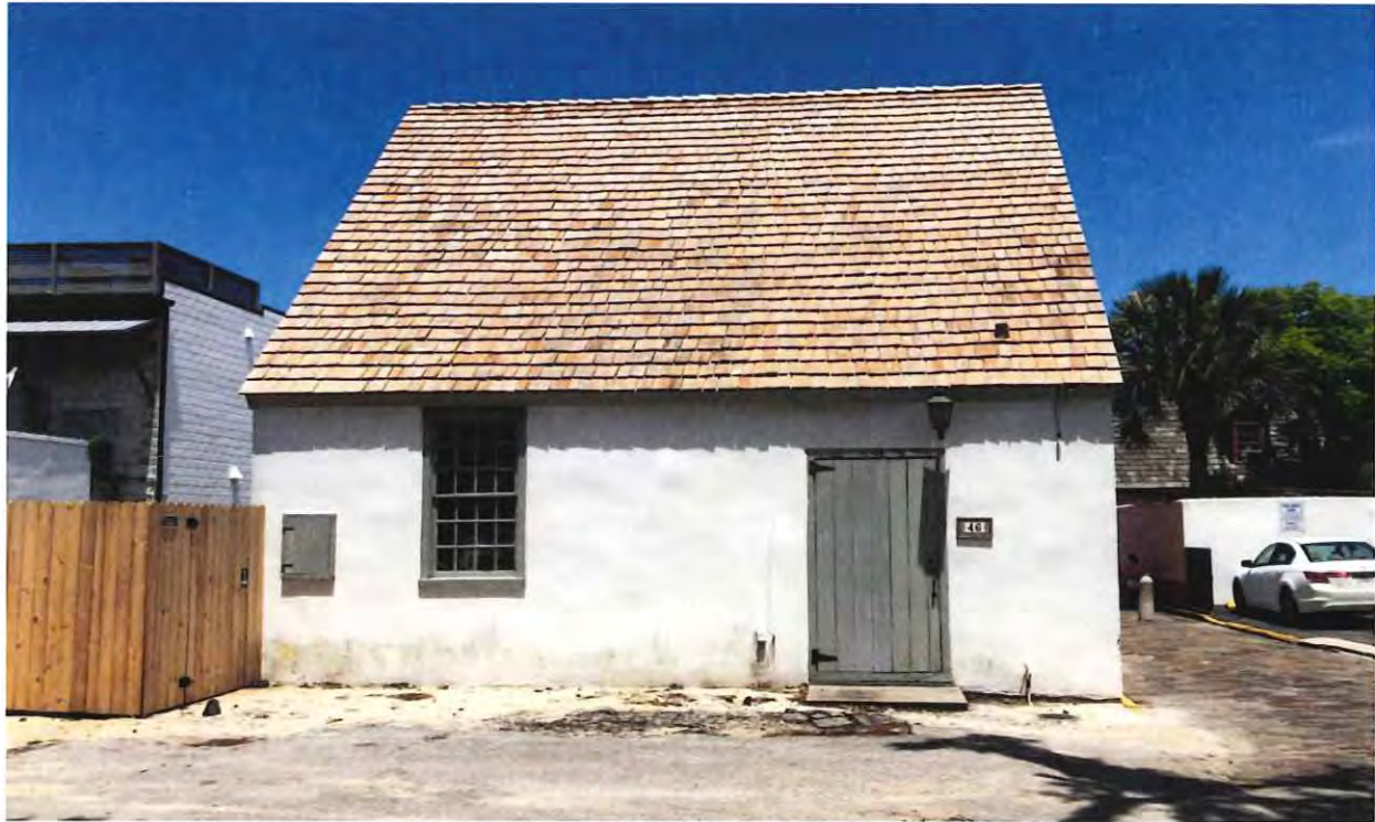
Existing Site Conditions on West Elevation
