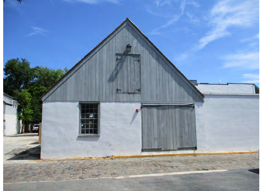
From Cuna Street, facing north (south elevation)
