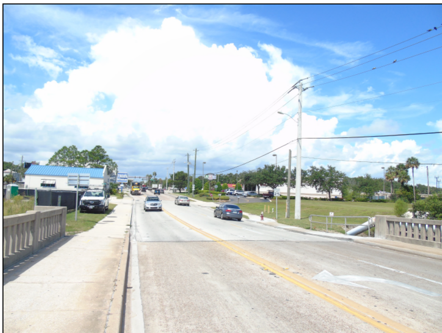
WEST APPROACH TAKEN FROM THE STRUCTURE
