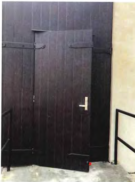
Existing Exterior Door at 48 King St.
