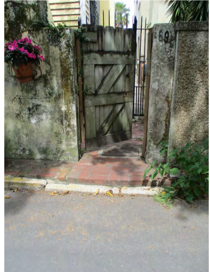
Front Façade / West Elevation and South Elevation with property walls and brick patio
