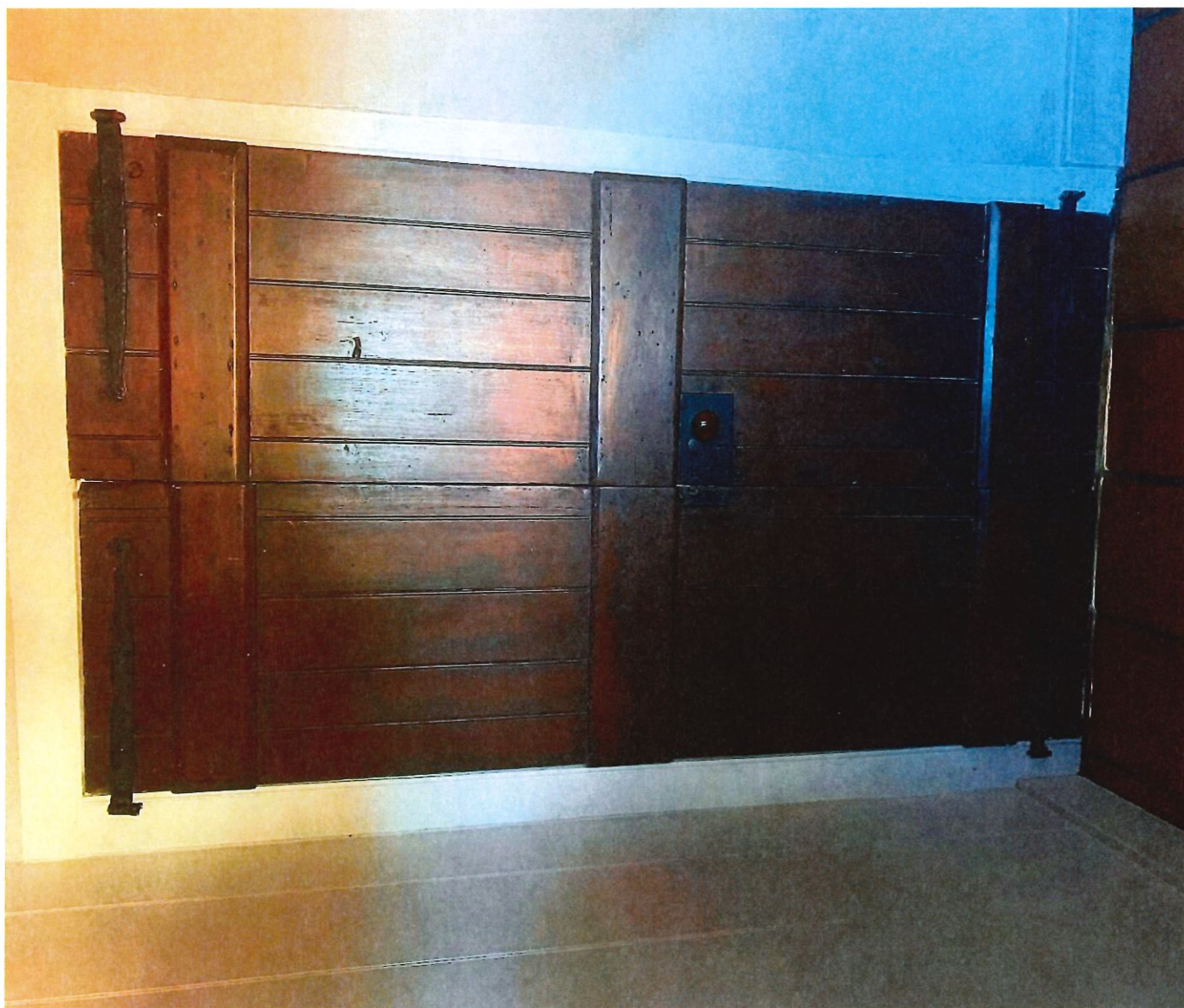
FIRST FLOOR, HABS STAIRHALL, AUGUST, 2020,, PHOTO 21 HABS DOOR #12, FACING WEST
