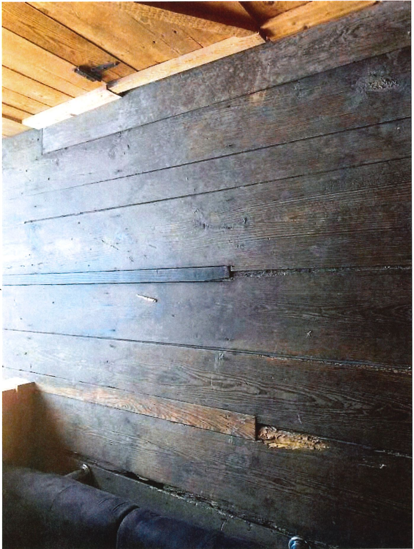
ATTIC, AUGUST, 2020, PHOTO 45 FLOORING, FACING SOUTH
