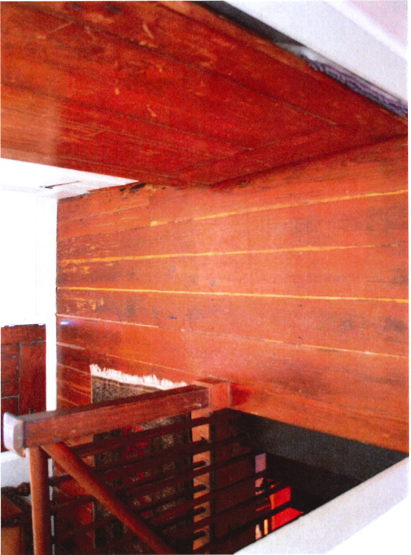
SECOND FLOOR, HABS STAIRHALL, AUGUST, 2020, , PHOTO 27 FACING EAST
