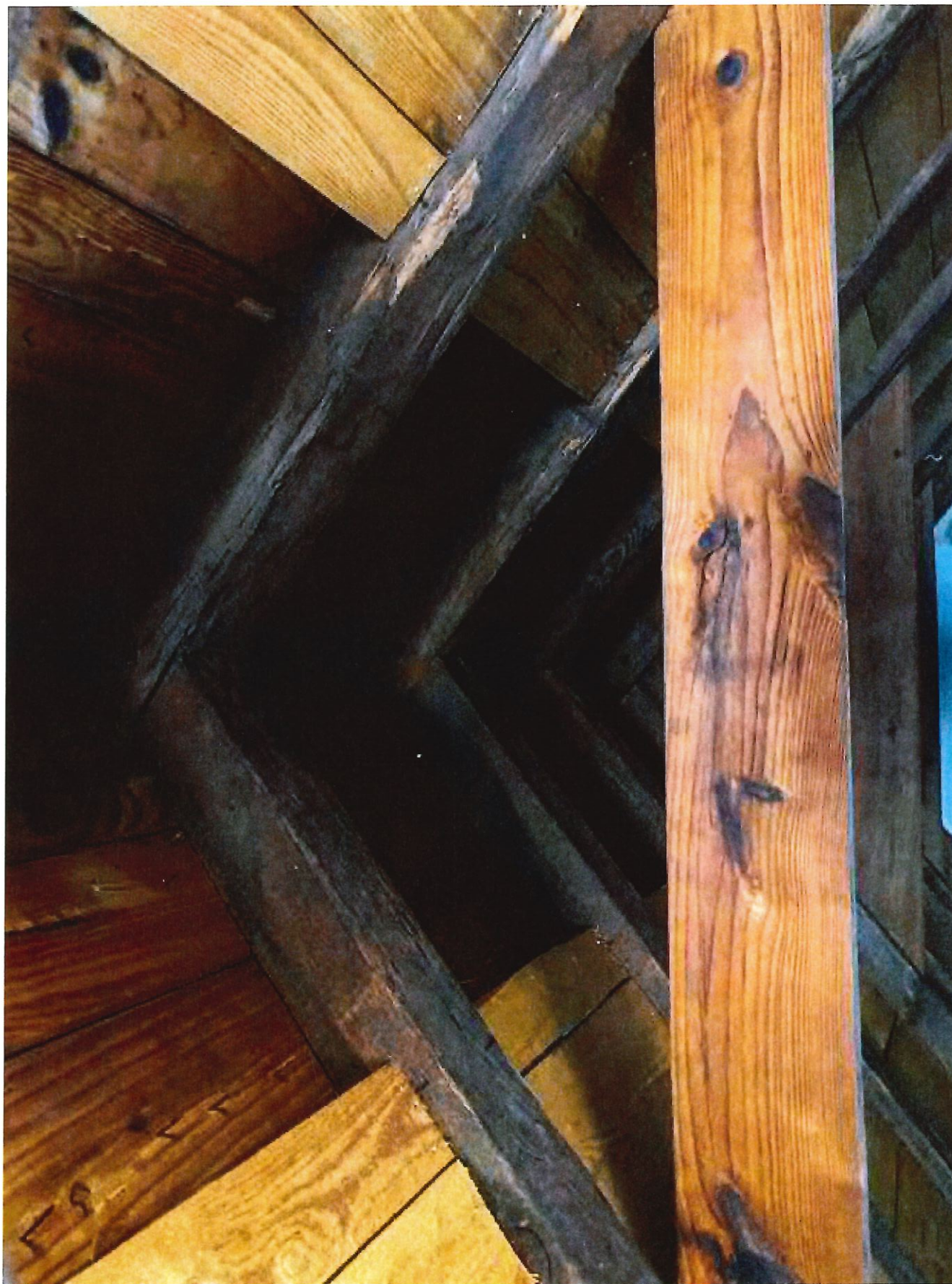
ATTIC, AUGUST, 2020, PHOTO 44 TRUSSWORK, DOWEL, FACING SOUTH
