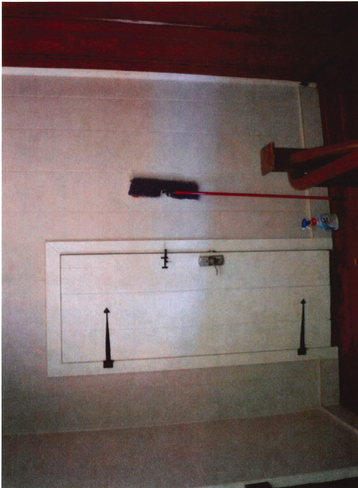
SECOND FLOOR, HABS STAIRHALL, AUGUST, 2020, , PHOTO 25 HABS DOOR #8, FACING SOUTH
