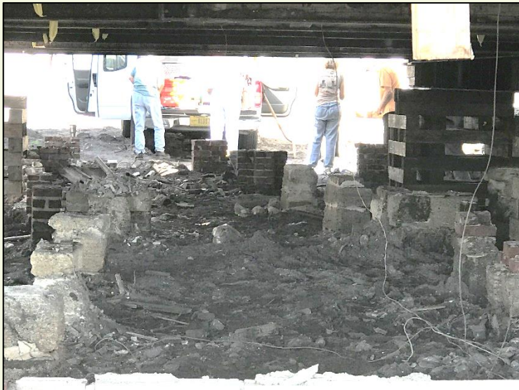
Archaeological investigation of foundation work
