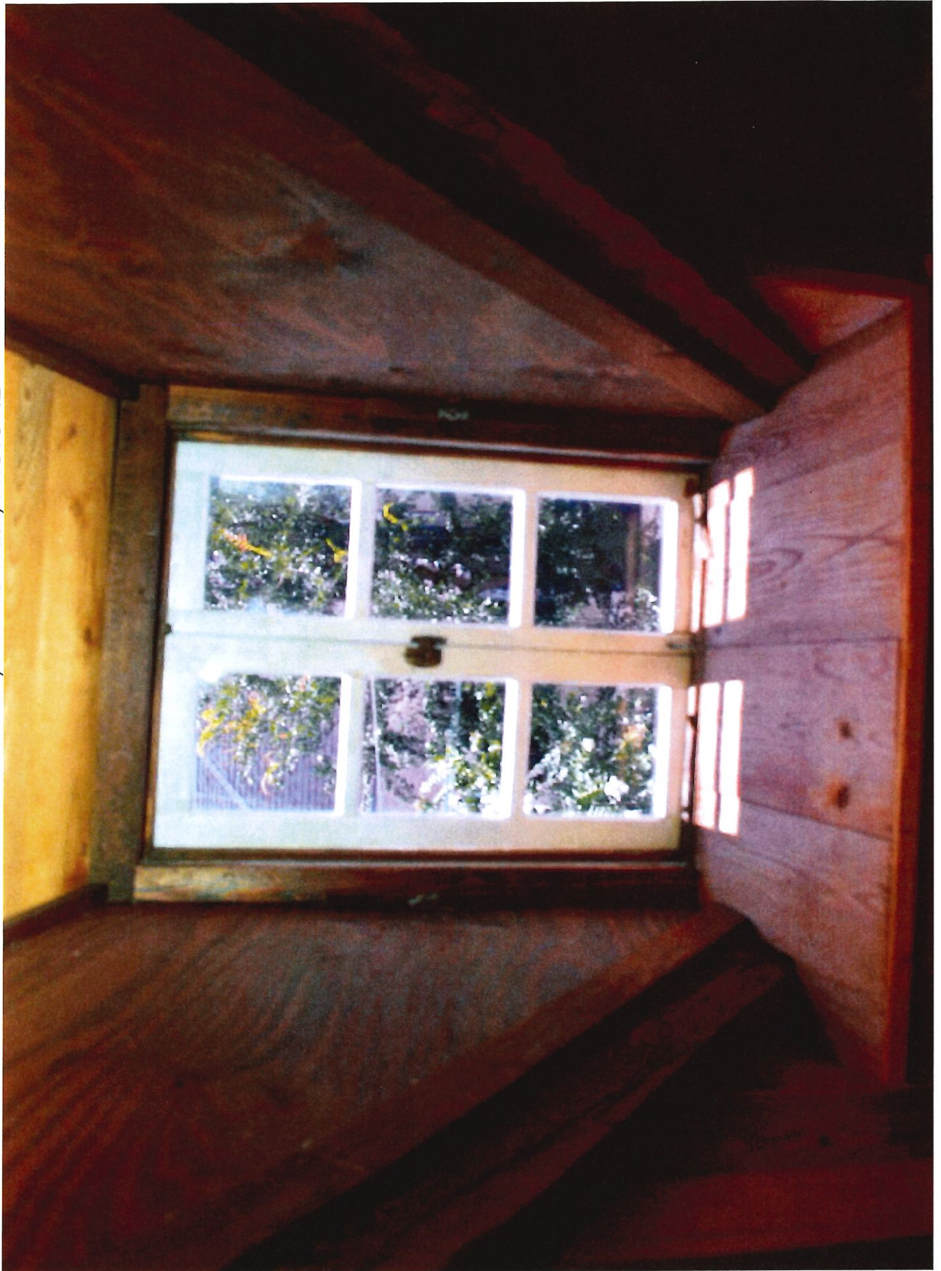
ATTIC, AUGUST, 2020, DORMER WINDOW, FACING WEST, PHOTO 42
