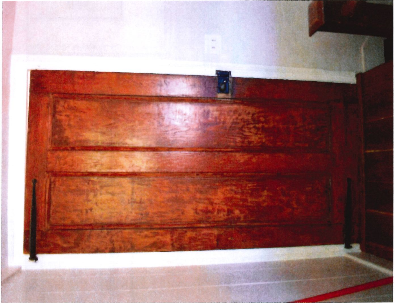
SECOND FLOOR, HABS STAIRHALL, AUGUST, 2020, , PHOTO 28 HABS DOOR #7, FACING WEST
