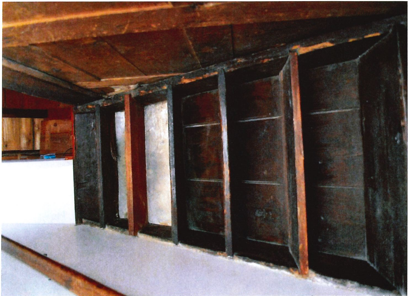
STEPS LEADING TO ATTIC, AUGUST, 2020, PHOTO 40 FACING WEST
