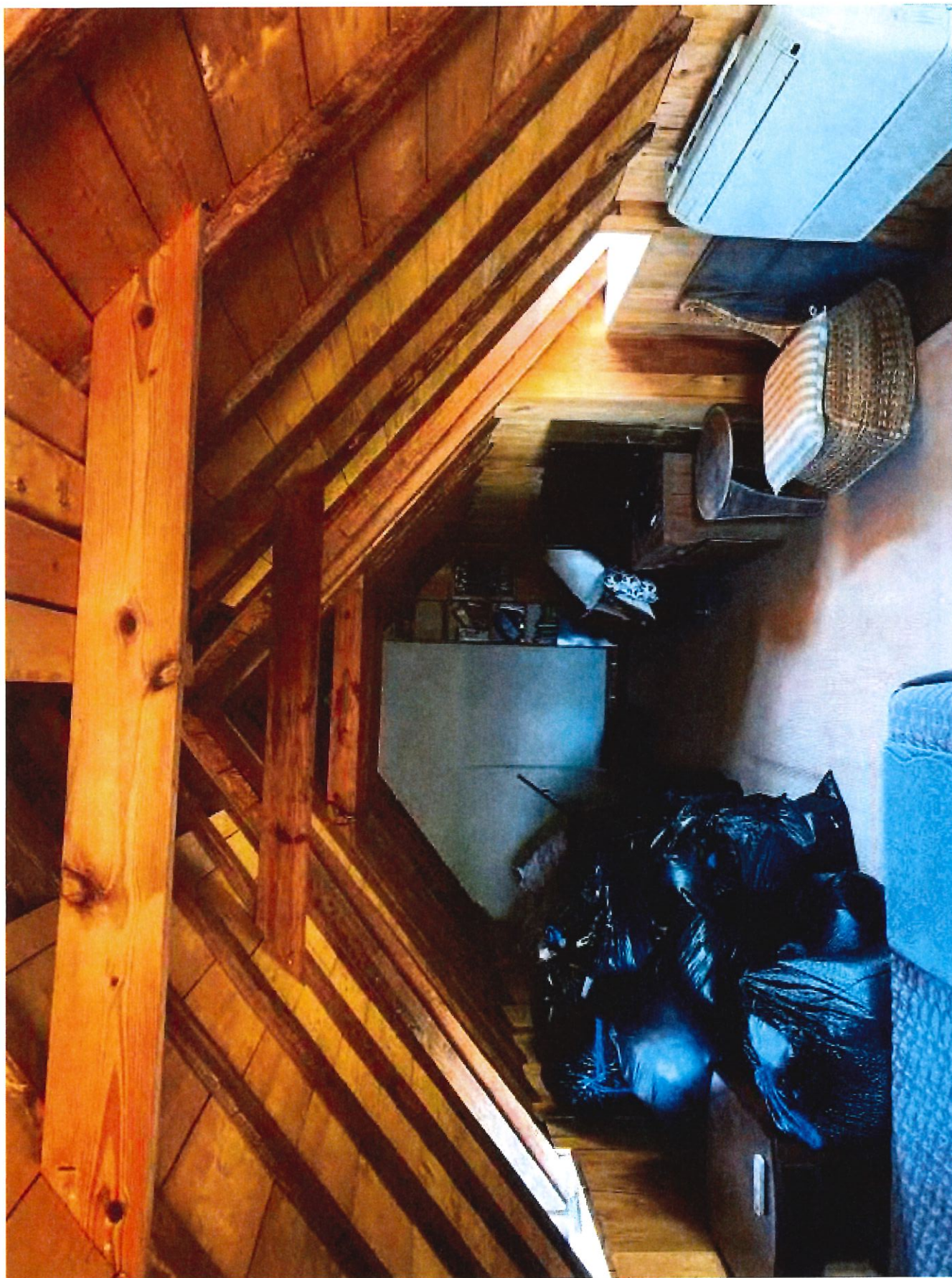
ATTIC, AUGUST, 2020, PHOTO 41 TRUSSWORK, FACING SOUTH
