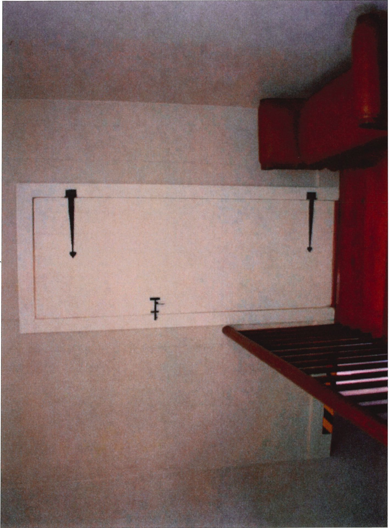
SECOND FLOOR, HABS STAIRHALL, AUGUST, 2020, , PHOTO 24 HABS DOOR #8, FACING NORTH
