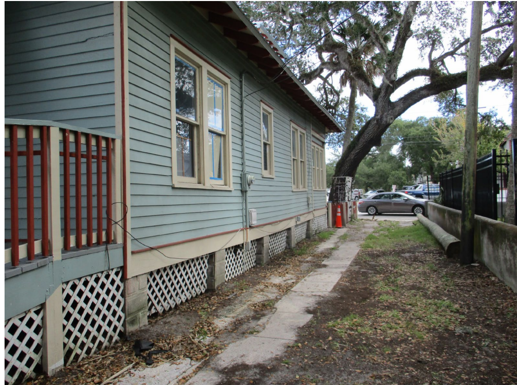
Along South Elevation, Looking East: Area of proposed addition and decking
