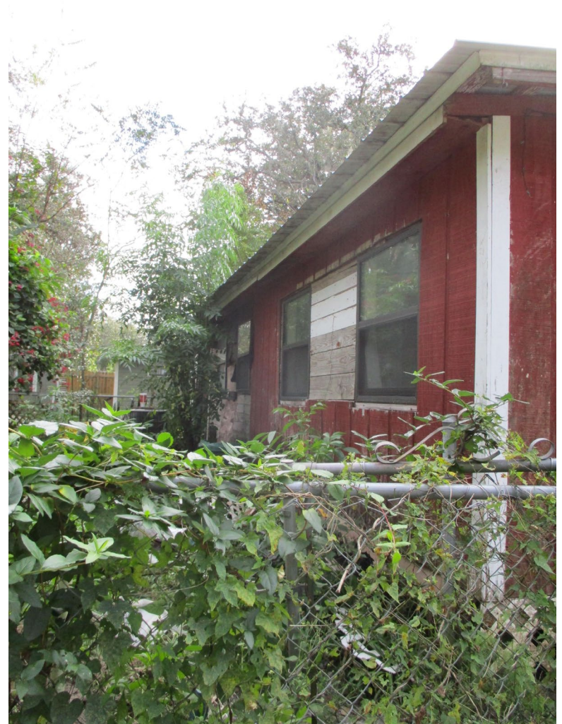
From Northeast corner and East Elevations
