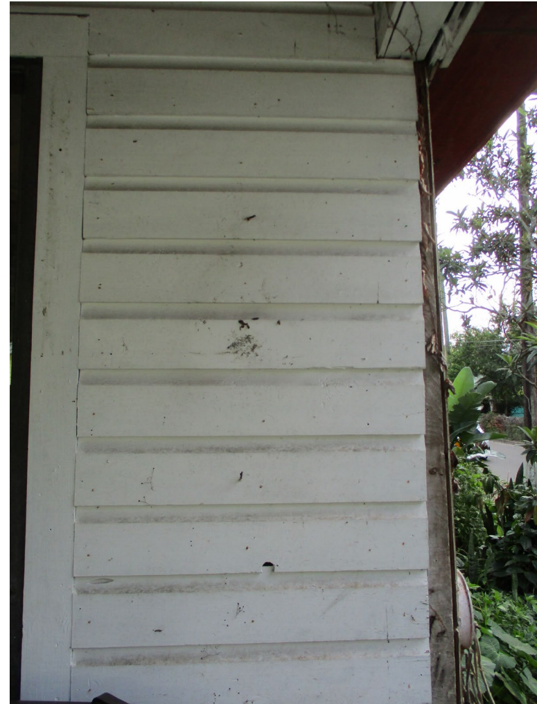
Northwest Elevations off corner of Phillips and Sidney Street / Drop siding on front façade
