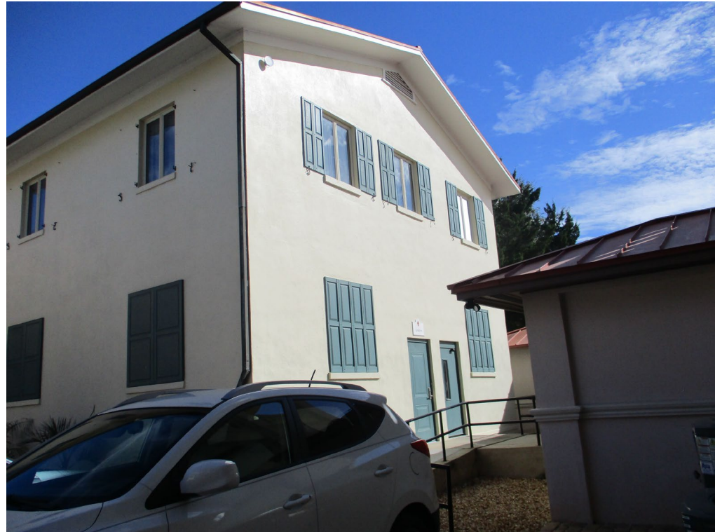
West and North Elevations
