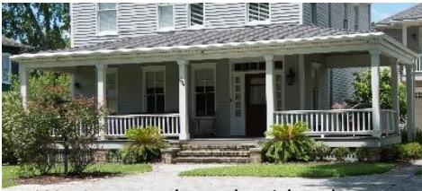
Wrap-around porch with columns and balusters
