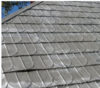
Stamped metal shingle roof
