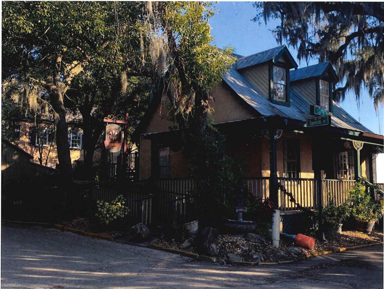
Photo 1.02 – View from Cuna Street looking northeast
