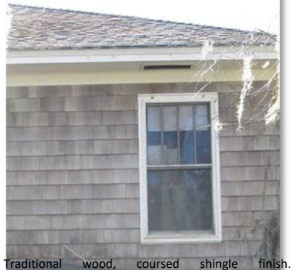
Traditional wood, coursed shingle finish. Changing the shingle pattern to a staggered design would change the character of the historic building from Shingle Style to a Bungalow or Arts and Crafts style.
