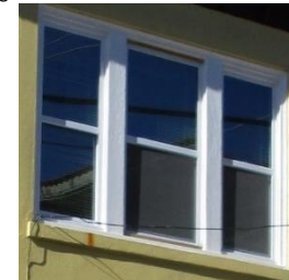
Original 3/1 and 4/1 lite vertical sash windows replaced with 1/1 across the entire building and would now require HARB approval if the building is designated historic.
