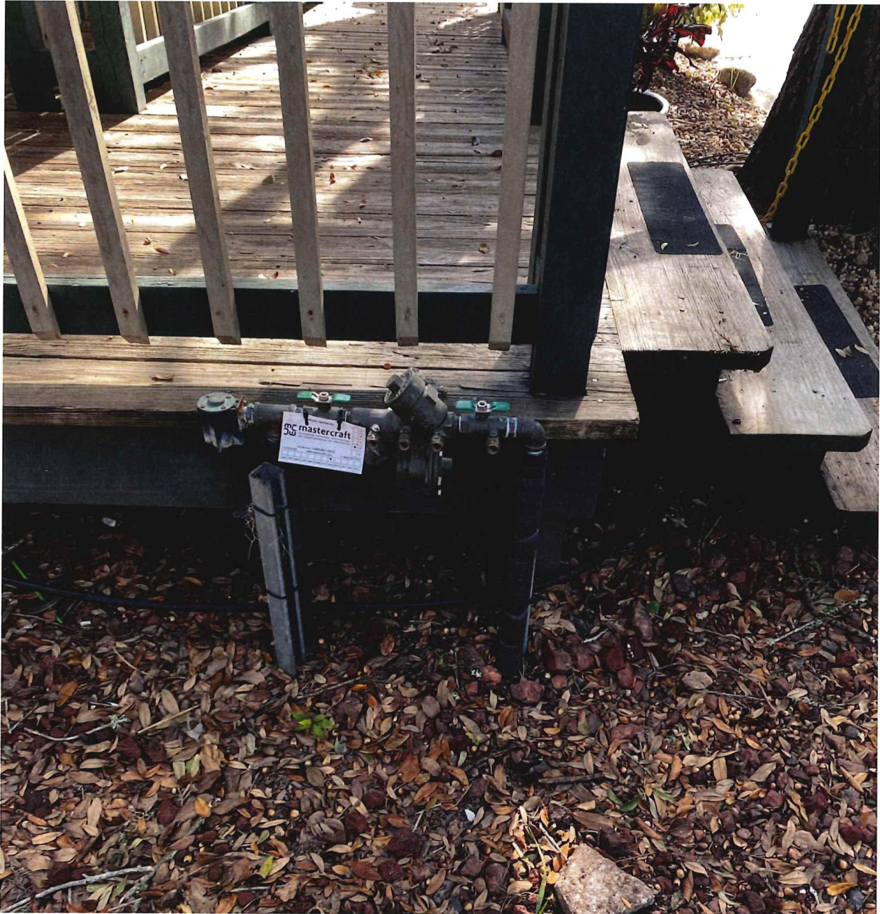
Photo 1.07 – Deck detail at far northwest end. Backflow preventer (to be relocated)
