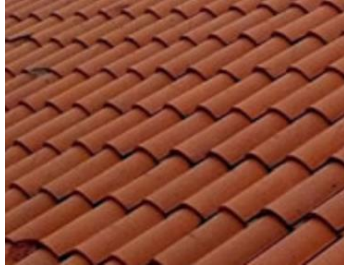
Clay tile roof
