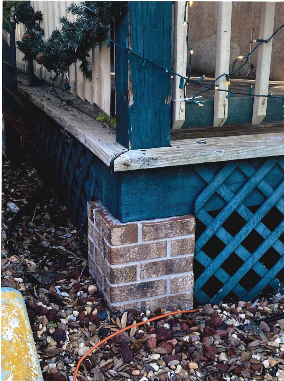
Photo 1.06 - Detail of existing porch column, rail, and pier foundation
