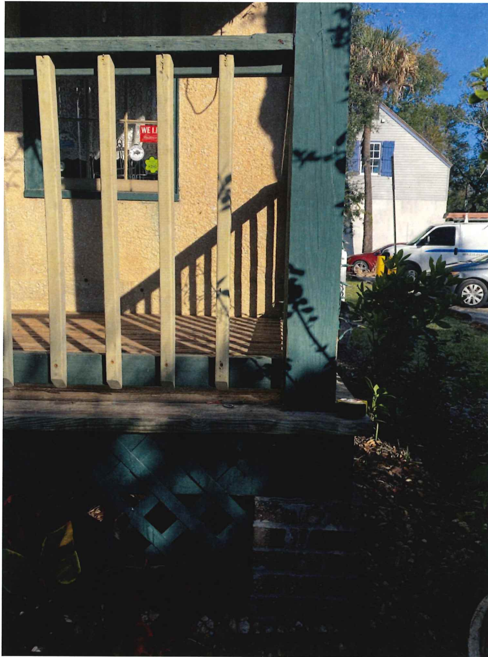
Photo 1.05 – Detail of existing porch column, rail, and pier foundation
