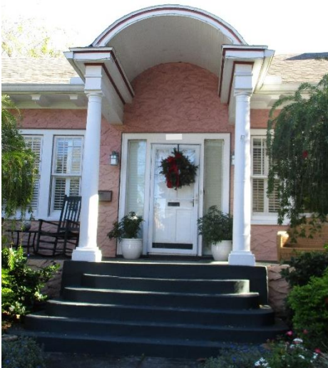
Central arched portico and stoop with decorative trim
