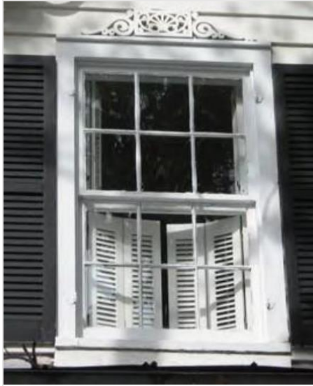
Traditional wood, vertical sash window with a 6/6 lite pattern
