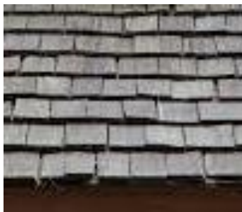
Wood shingle roof
