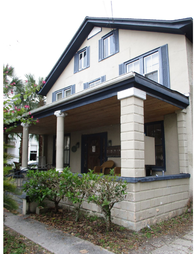
Front Façade / East Elevation: Smooth Plaster on front with different windows visible
