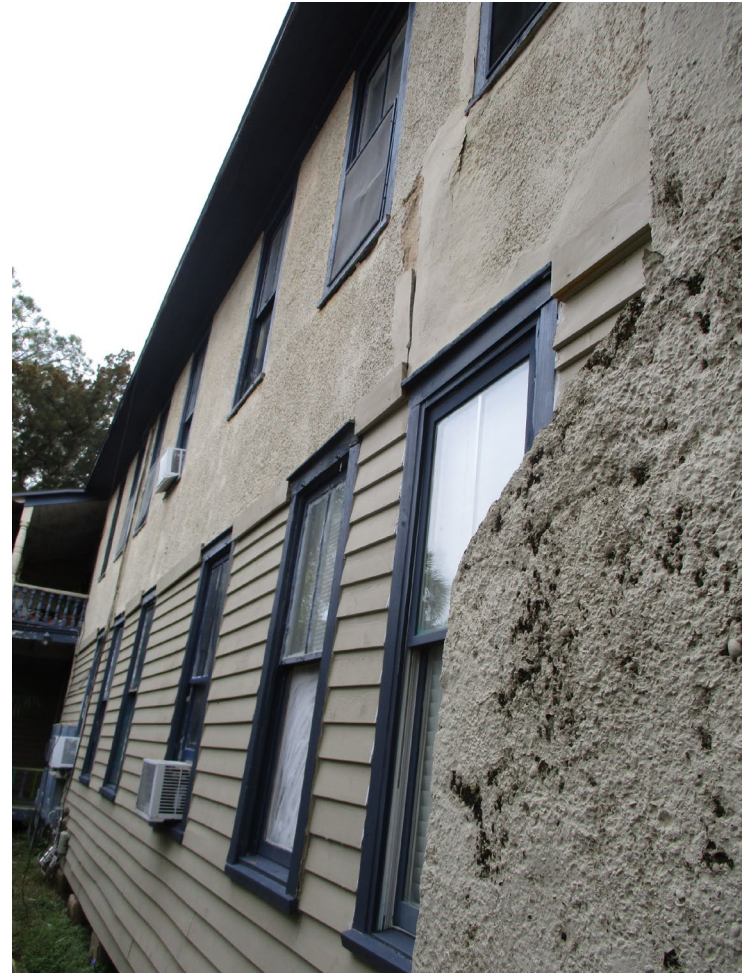
South Elevation: East of remaining original side porch
