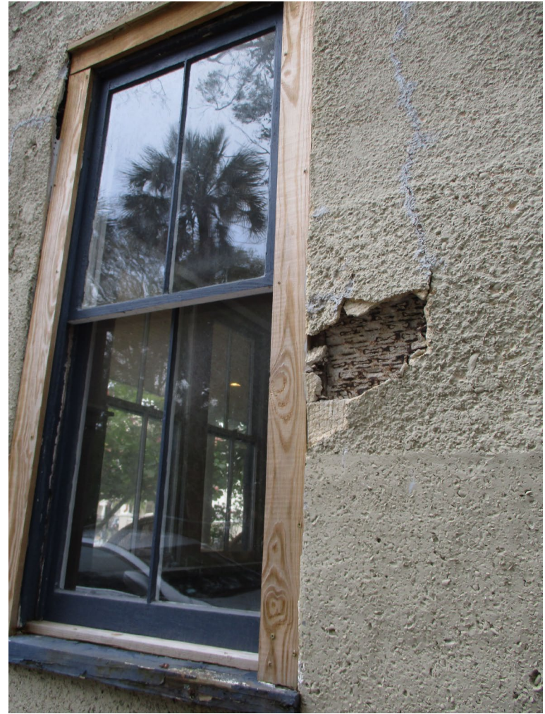
North Elevation: plaster
