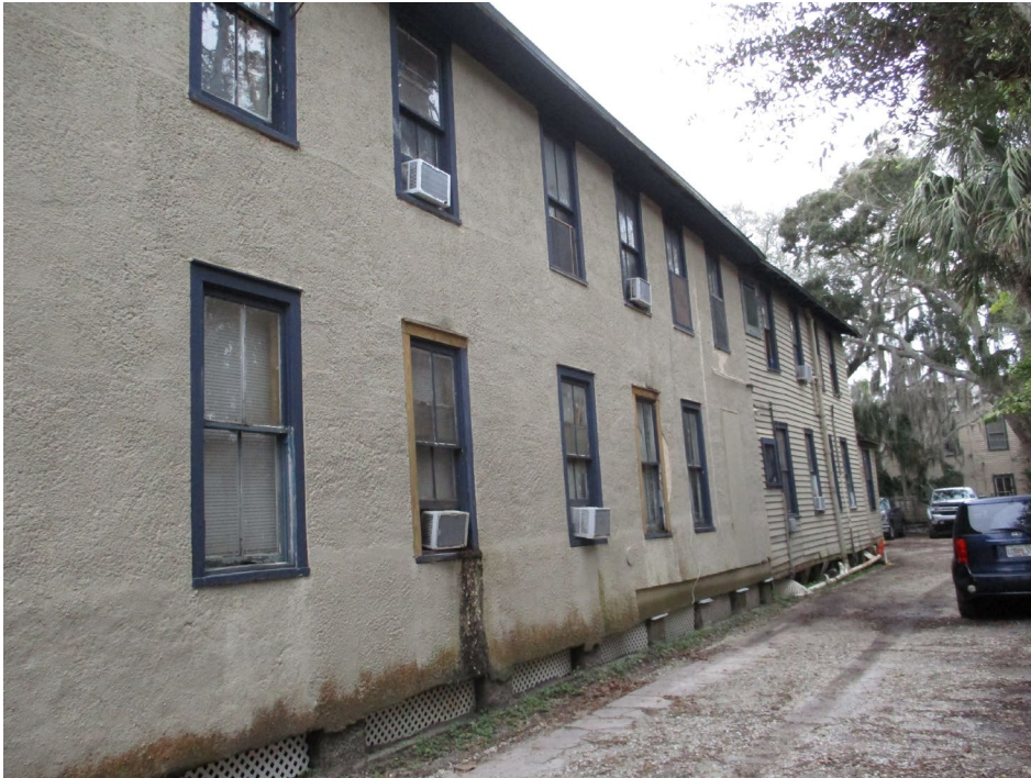
North Elevation: Plaster on front/east end with different wood siding and windows visible
