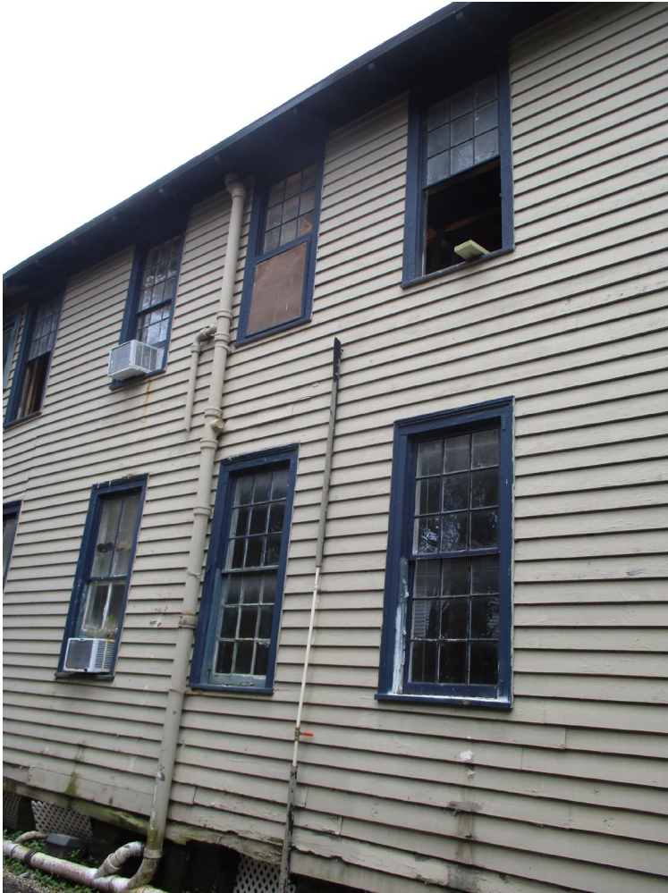
North Elevation, toward rear: different wood siding and windows visible
