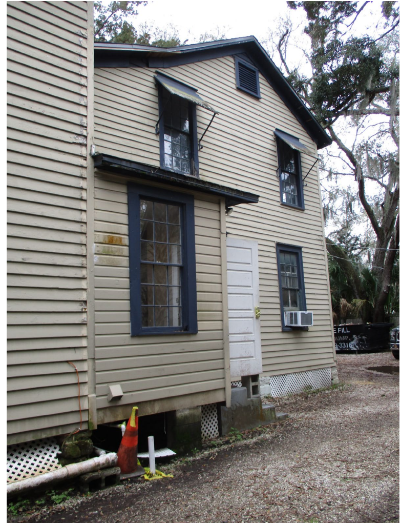
North Elevation, toward rear: different wood siding and windows visible
