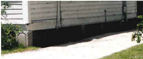
Coquina concrete block is a material unique to St. Augustine
