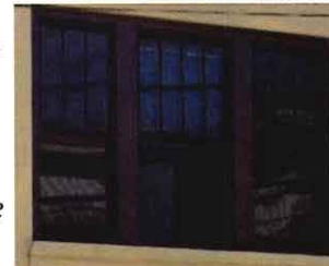
Original 3/1 and 4/1 lite vertical sash windows replaced with 1/1 across the entire building and would now require HARB approval if the building is designated historic.
