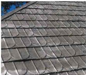
Stamped metal shingle roof
