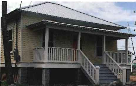
New front porch at the elevated floor height matching the historic character
