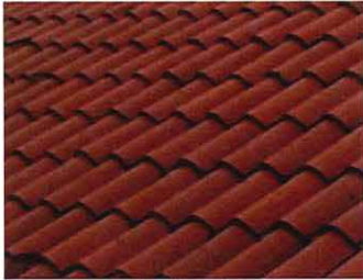
Clay tile roof
