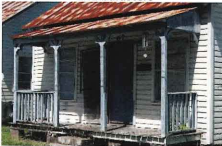
Centered porch with turned balusters and folk-style bracketed posts
