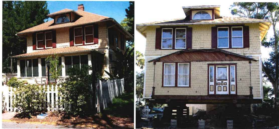
Foundation (and porch) was removed to allow for the building to be elevated to a new floor height for a flood mitigation project.
