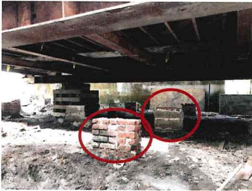
A building elevation project revealed unique coquina stone piers (background) along with traditional brick piers (foreground)
