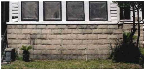
Coquina concrete block is a material unique to St. Augustine
