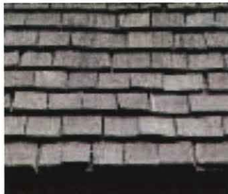
Wood shingle roof
