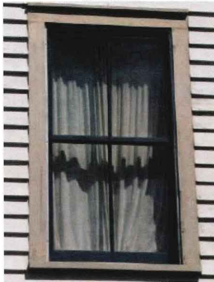
Traditional wood, vertical sash window with 2/2 lite pattern
