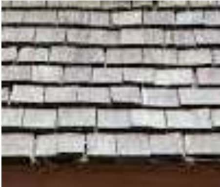
Wood shingle roof
