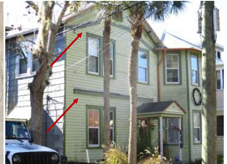
Evidence on the Sanborn map (left) and the building shows there used to be a historic two-story frame porch likely removed ca. 1930-1950s when asbestos siding was added. Reconstructing a compatible porch could be approved by staff.
