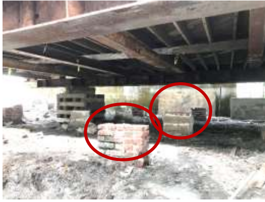
A building elevation project revealed unique coquina stone piers (background) along with traditional brick piers (foreground)
