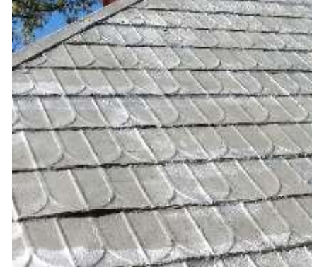
Stamped metal shingle roof
